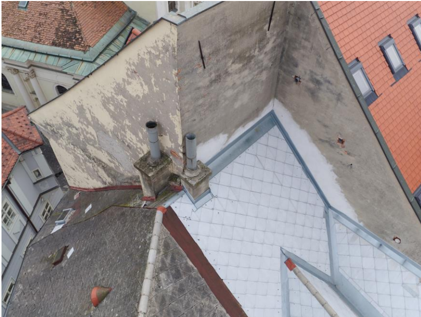
Revision of hardly accessible chimney
