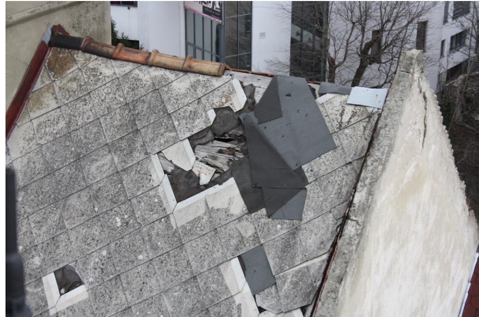
Aerial inspection of the roof
